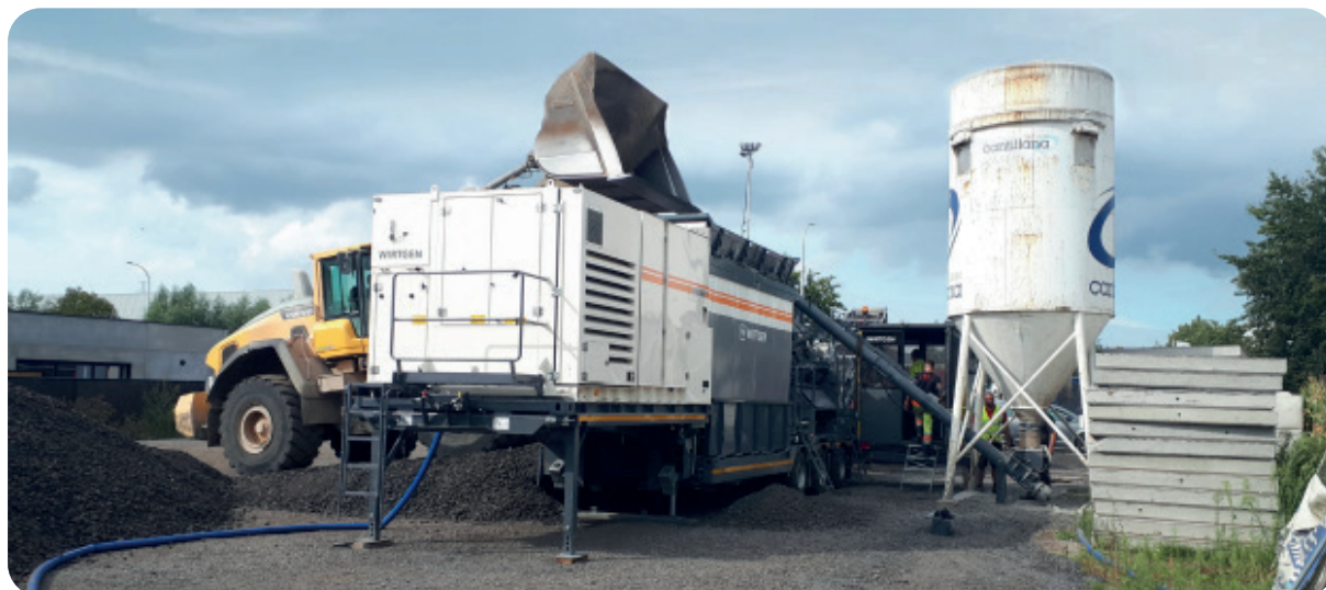
Installation de bitume moussant
